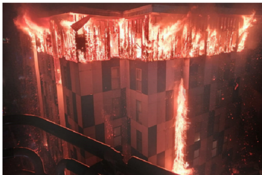
The Cube, a student block in Bolton, was covered in high-pressure laminate cladding
