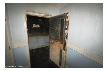
2.7 The escape staircase, which was constructed to provide protection for those escaping from the building, remained largely undamaged.
