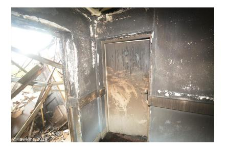
2.5 The photograph above shows the condition of the wall in a flat on the "fire" side of the corridor. Through the doorway to the left, the flat has been completely destroyed by the fire, while the corridor, although damaged, remained in place. The walls around the corridor were required to provide 60 minutes' fire protection, and they largely appear to have done so.
