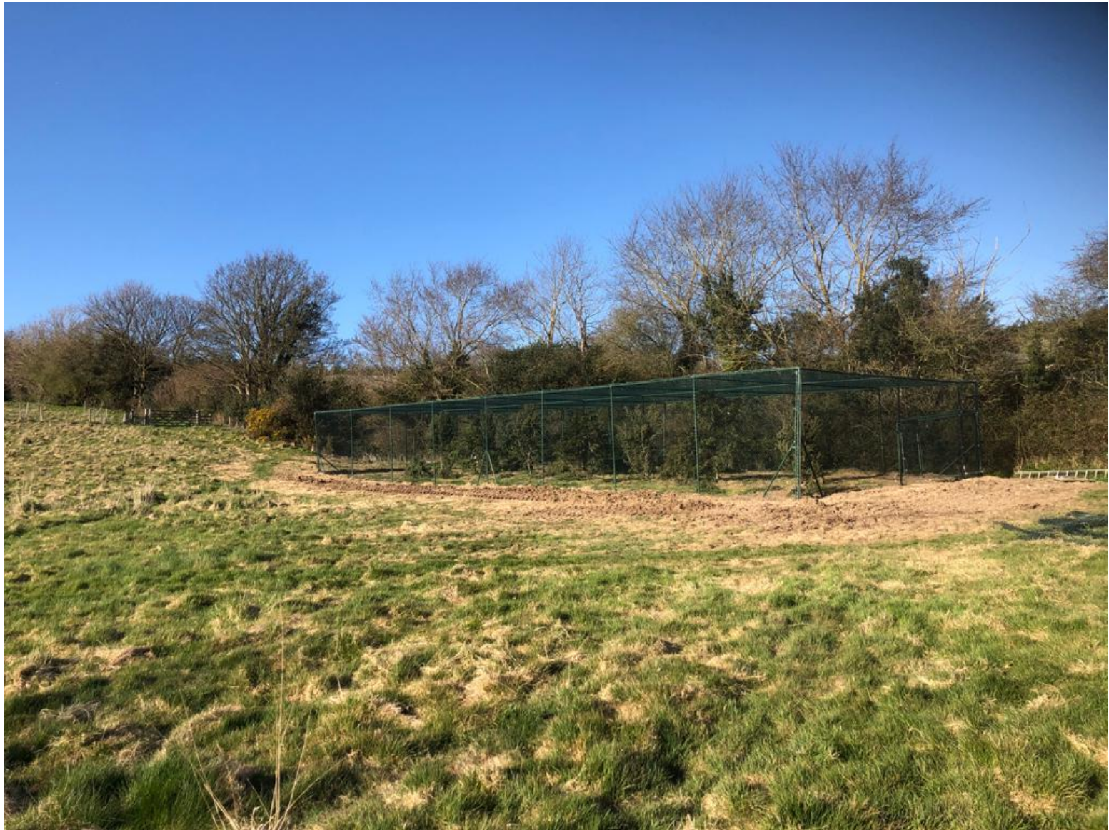
Rehabilitation enclosure, measuring around 85 ft by 29ft wide by 10ft high, containing natural vegetation. Completed in April 2021
